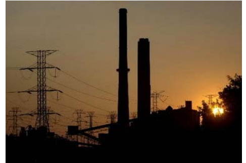
Jamie-Andrea Yanak, Associated Press FirstEnergy Corp.'s Eastlake power plant
