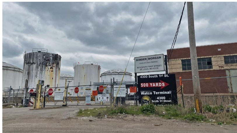
Kinder Morgan’s facility on the banks of the Mississippi in Dutchtown St. Louis
